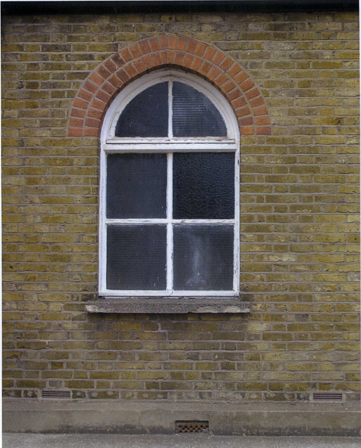
3. From Car Park; typical Window to North Hall
