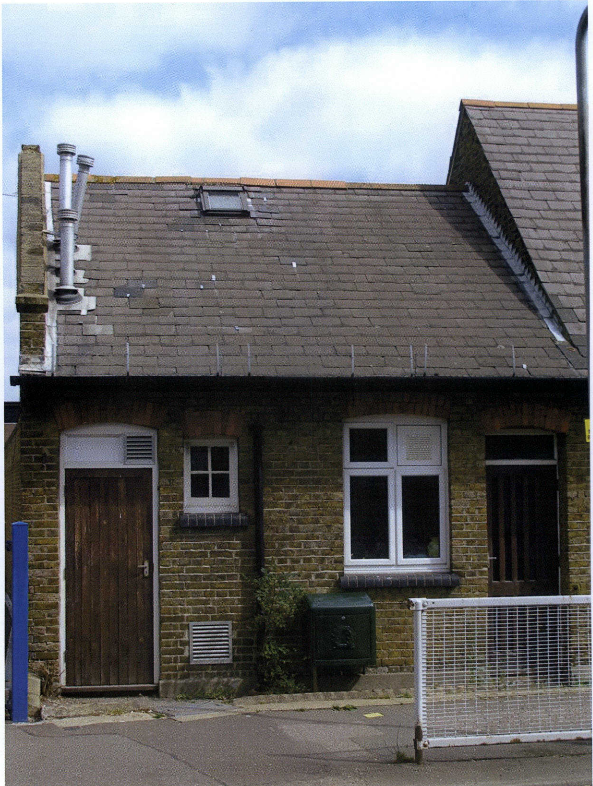
8. Rear Kitchen Building; Love Lane Elevation
