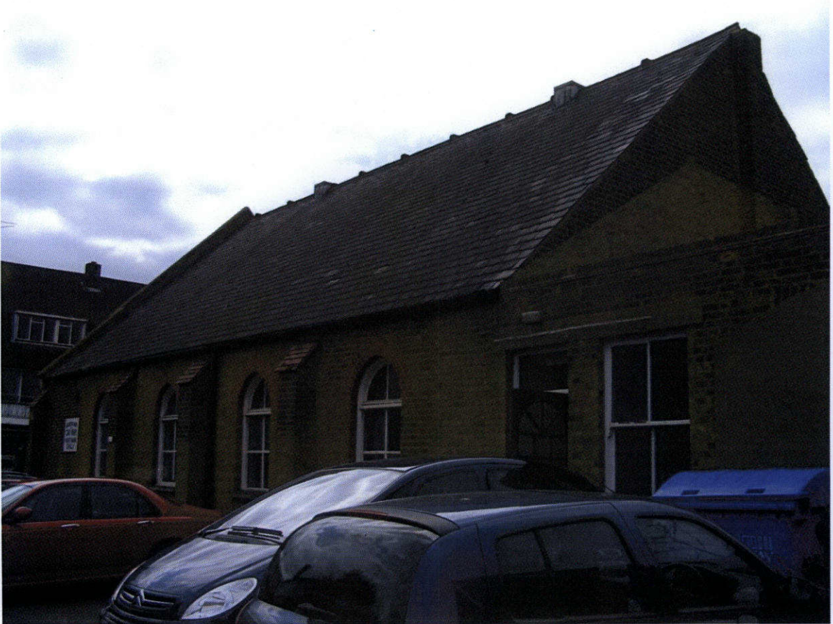
1. From car park; looking South East.
