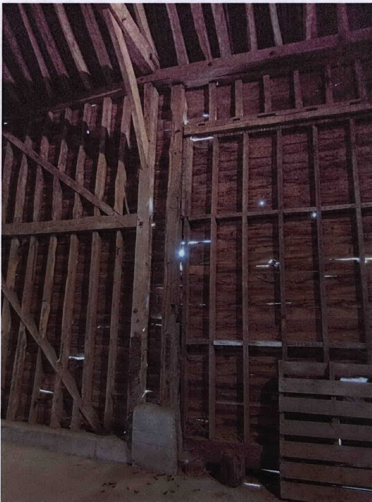
Figure 14 - former double, full height door infilled with a later panel
