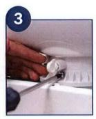
Attach the Greenstar Xtra to the adaptor using the included unit fixing screw.
