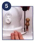
Fit the horizontal or vertical flue adaptor into the Greenstar Xtra flue connection point. Secure the unit with the three fixing screws provided.
