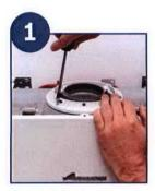
Dissemble the adaptor from the Greenstar Xtra by removing the front fixing screw. Using the three screws provided secure the adaptor to the boiler.
