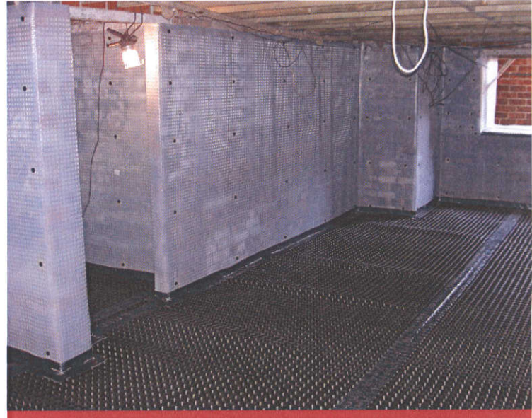
TYPICAL WALL/FLOOR DETAIL BELOW GROUND
