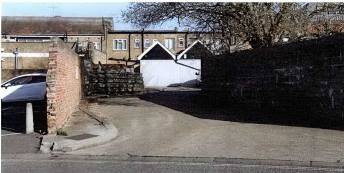
The Smile Centre on the left with access to the rear of 31 and lower numbers on right
