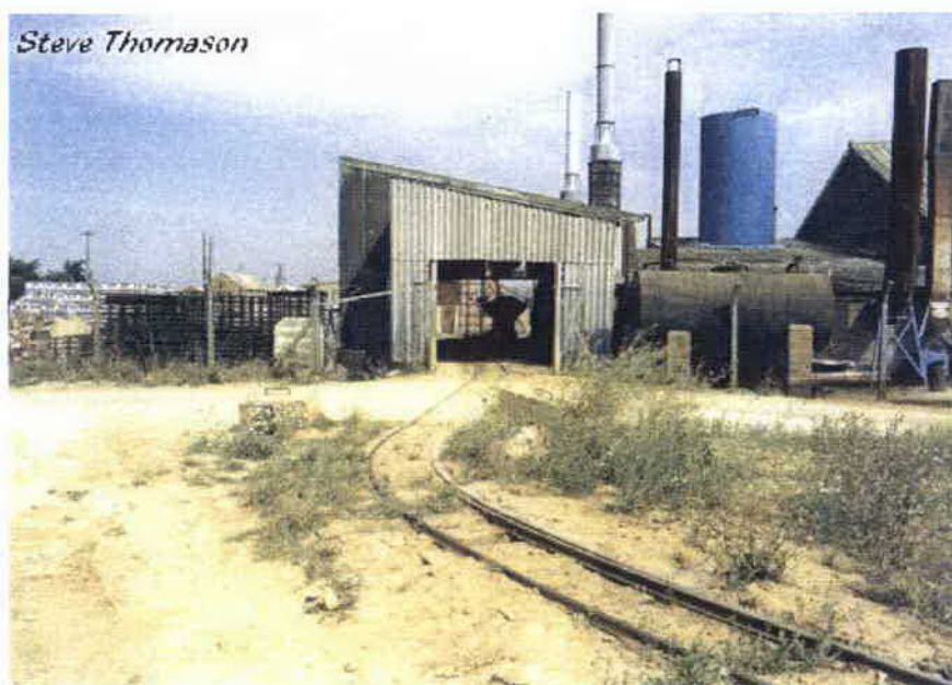
Illustration 10: narrow gauge railway bringing weathered clay to the tipping shed at the south side of the brickworks. The chimneys for the downdraught kilns can be seen in the background. © Steve Thomason http://www.inqr.co.uk
