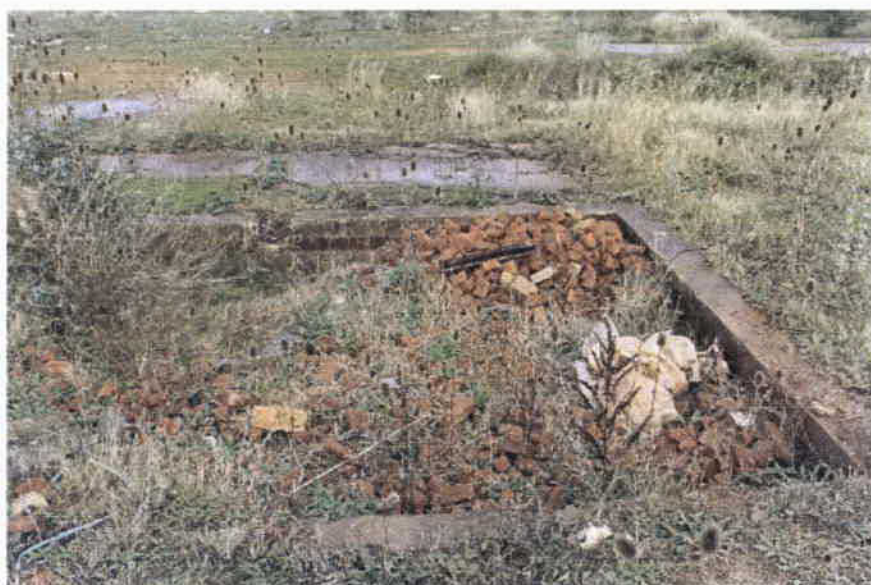
Illustration 12: rubble-filled flue pit , all that remains of the downdraught kilns.
