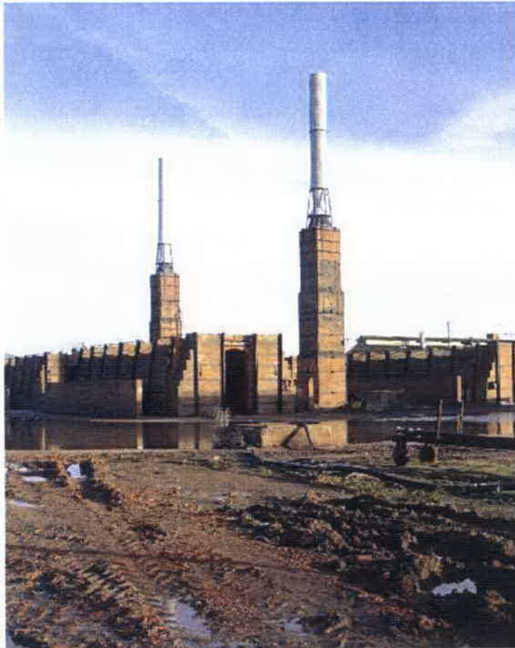
Illustration 9: chimney stacks between the pairs of downdraught kilns.
