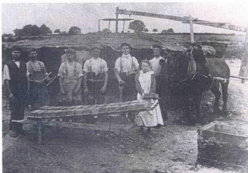
Illustration 3: a late Victorian brick yard in Chelmsford , with young workers (possibly related family members) standing in front of a horse-driven pug mill and with a barrow of hand-made bricks in the foreground. Similar scenes would have been found around the brick fields of Wakering.
