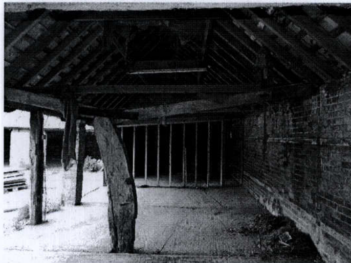
Photo 4: Interior of western building
