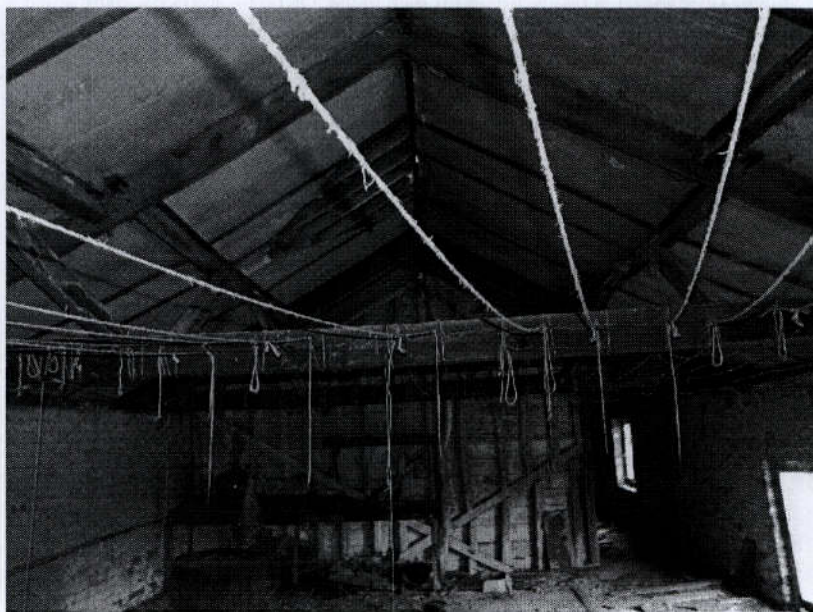
Photo 12: Upper floor of brick building – the roof is lined with plasterboard
