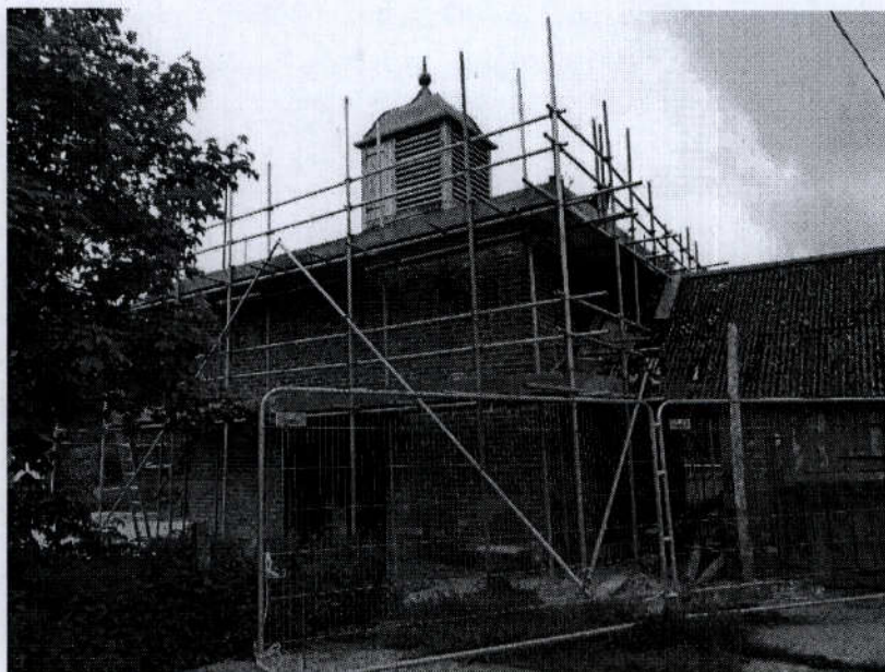
Photo 9: Dove cote building
