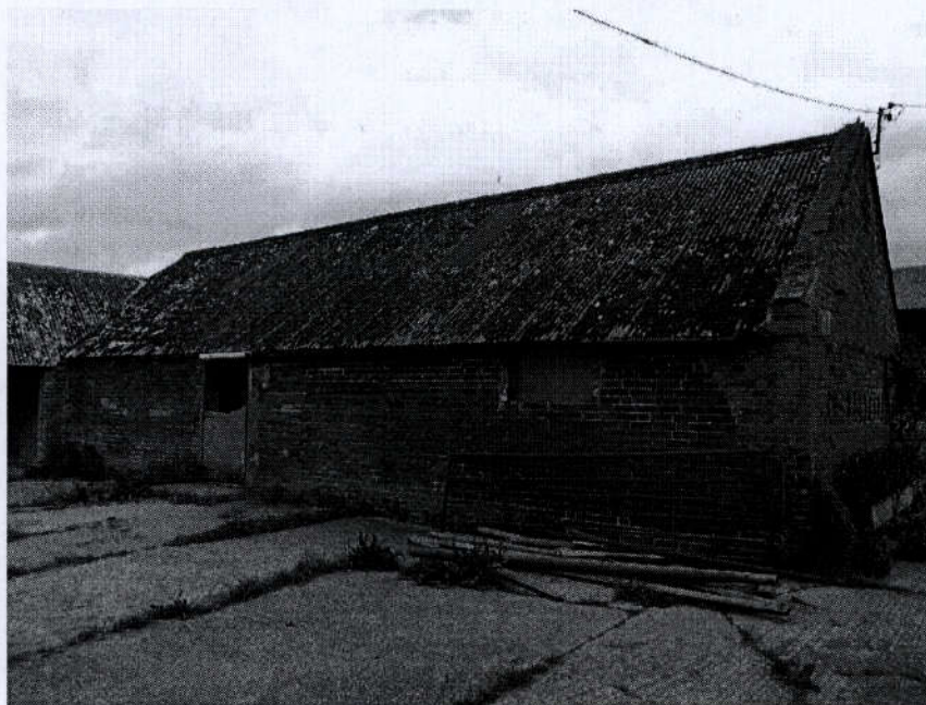
Photo 5: Former livestock shed on northern side of courtyard
