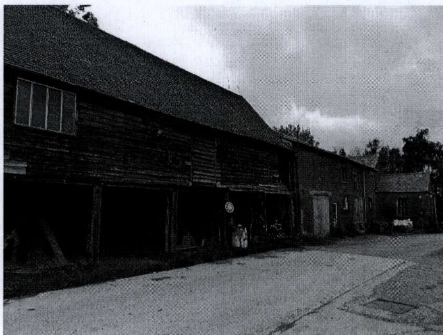
Photo 10: The cart lodge (with upper floor) and brick building
