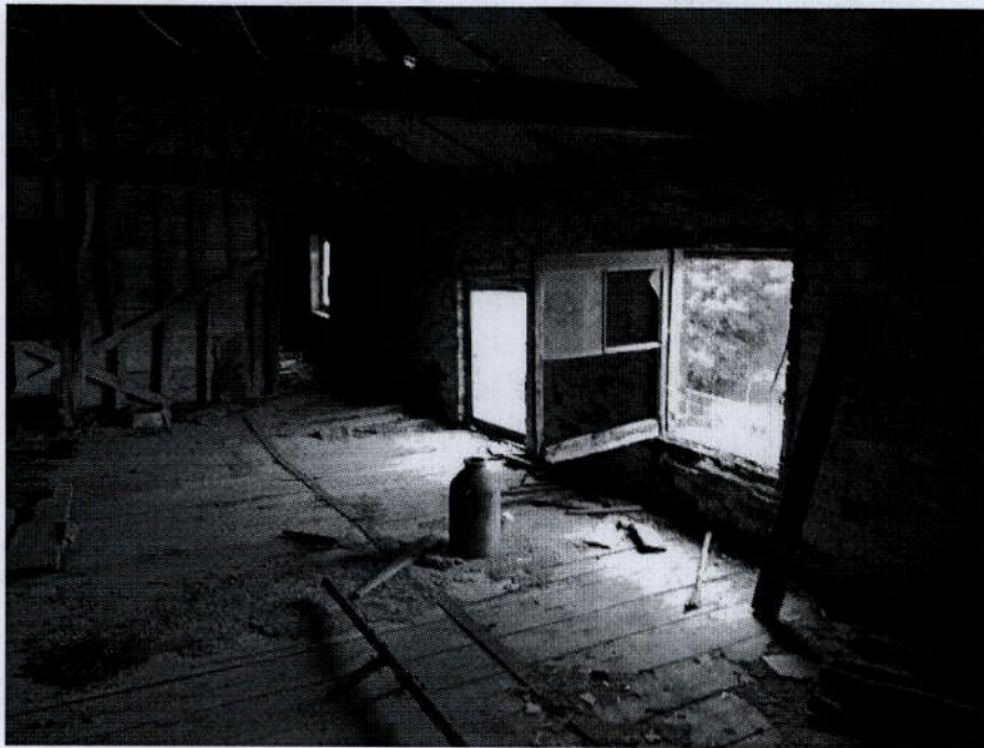
Photo 12: Upper floor showing missing windows
