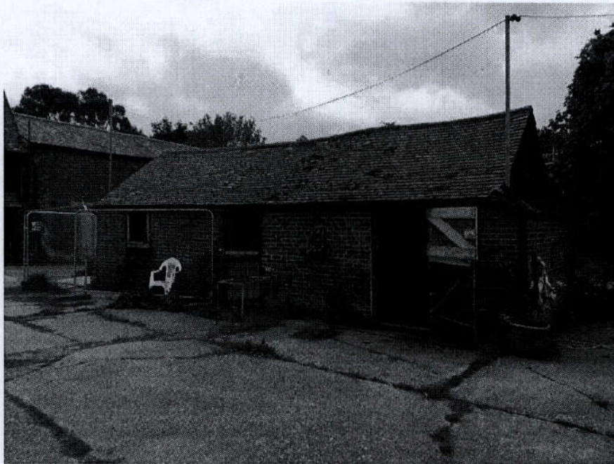
Photo 7: Stables due for demolition
