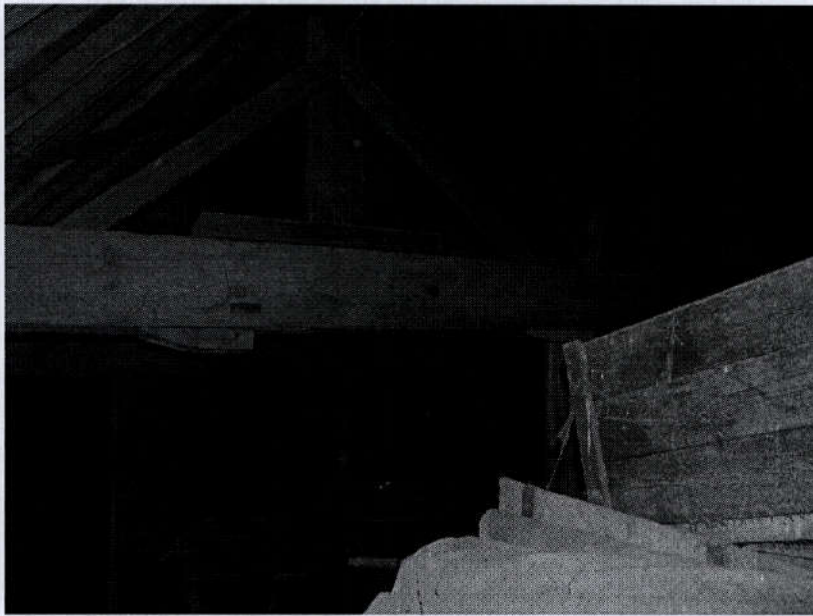
Photo 11: Upper floor of cart lodge
