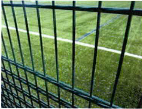
Example of rigid mesh ball-stop fencing panel (868 gauge)
