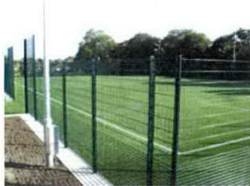
Example of ball-stop fencing
