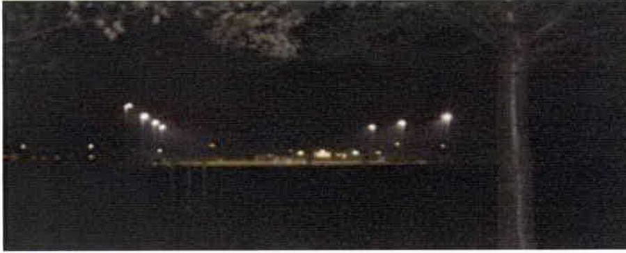
Example of floodlighting from the end of a full sized artificial sports pitch at night with an average 286lux floodlighting system from 50m away without screening.
