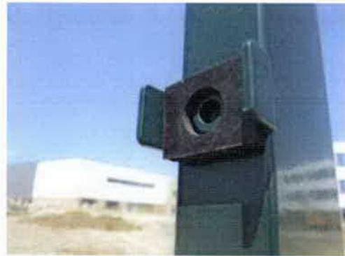
Example of neoprene washer within U shape fixing bracket
