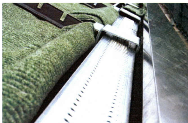
Internal Optigreen Drainage Conduit, with Structured Storage Fleece Type SSV 800 placed above
