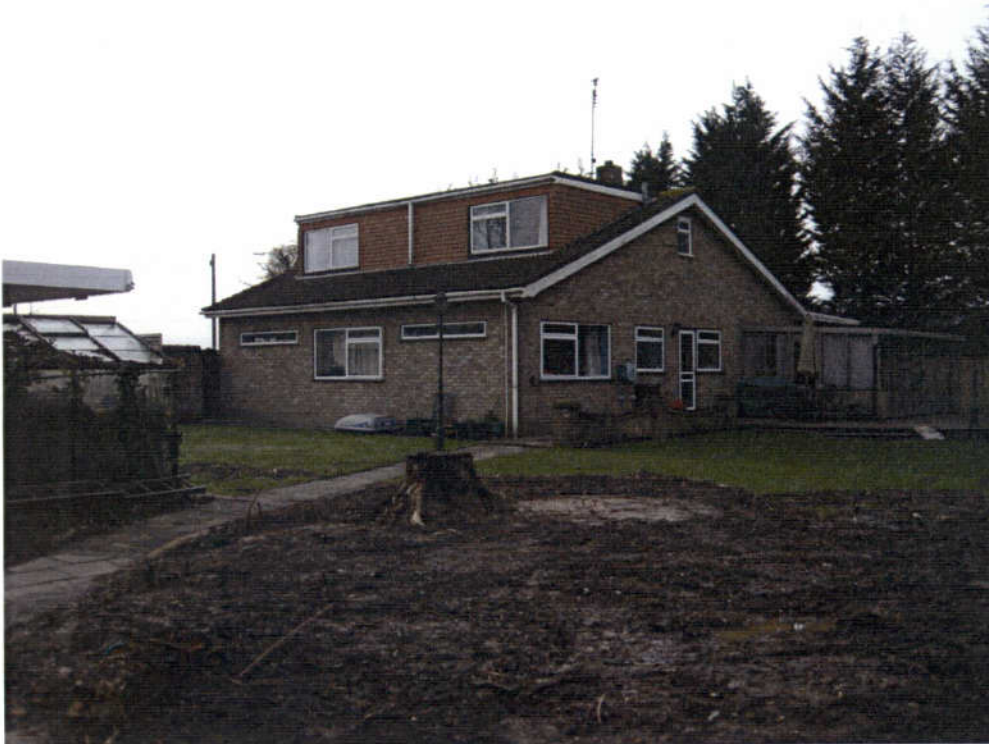
11.4 Site Photograph – 'Grange Villa' residence
