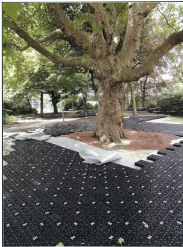
Figure 1. - Installed 'Arboraft' system around retained existing trees.
