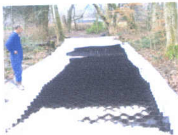
CellWeb during installation.
