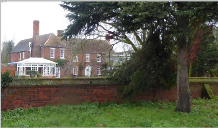
Plate 42. Brick coping and buttresses on S length of wall
