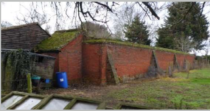
Plate 40. Outer face of W length of wall with buttresses
