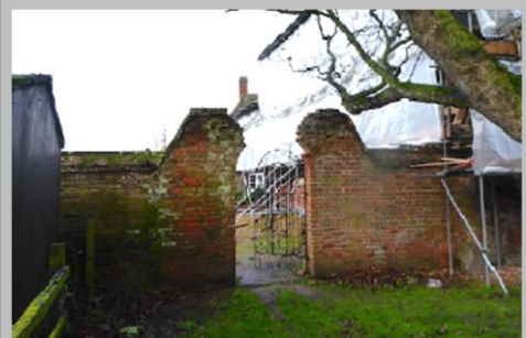
Plate 43. Collapsed arch in wall adjacent to cart lodge
