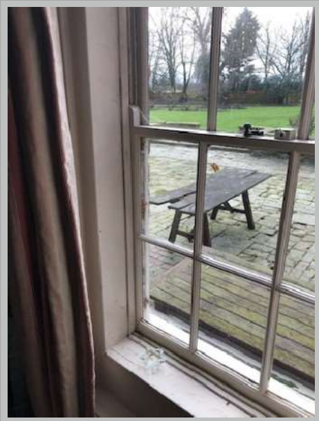
Plate 4a. Ovolo moulding on ground floor windows with horns
