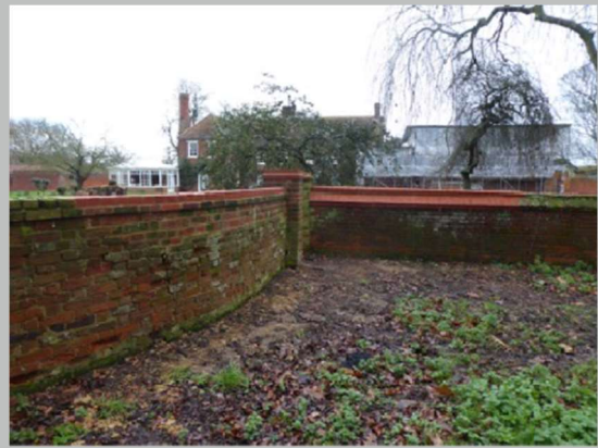
Plate 43. Repaired coping on S Length of wall
