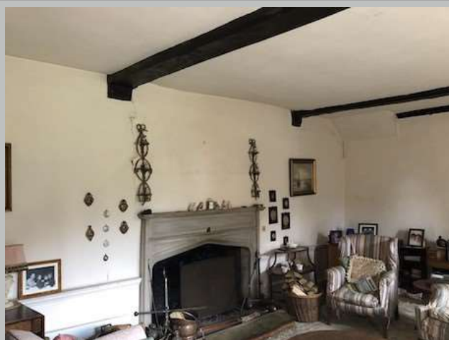
Plate 15. "Tudor-arched" fireplace and beams in hall/living room
