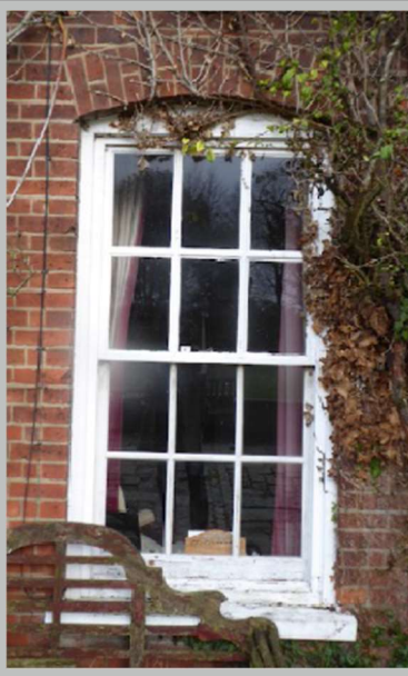
Plate 4. 6 over 6 box sash window without horns and with deep segmental brick head
