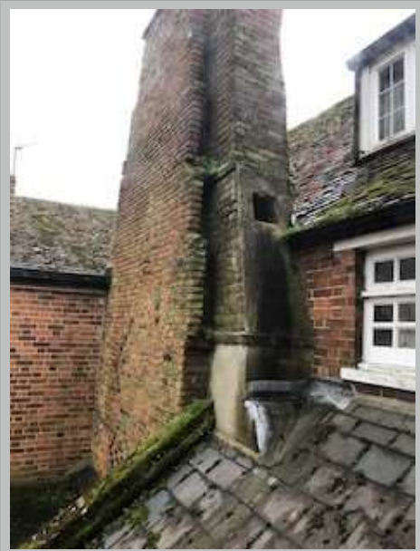
Plate 12. Chimney much-rebuilt
