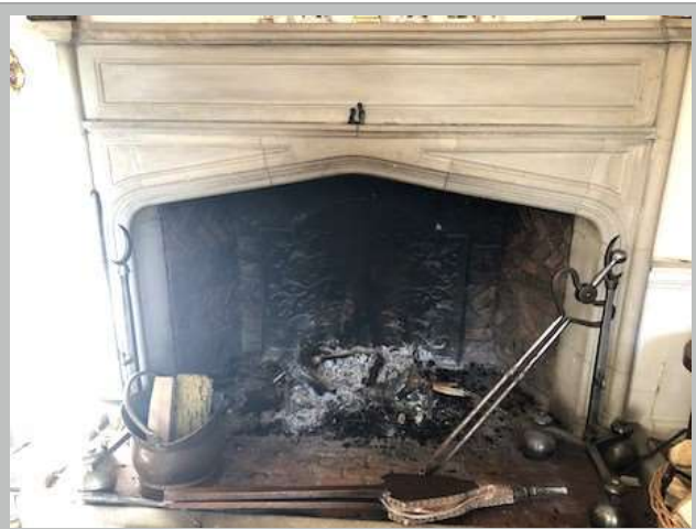
Plate 30. Edwardian Tudor style fire surround with CR/GR cast iron back plate
