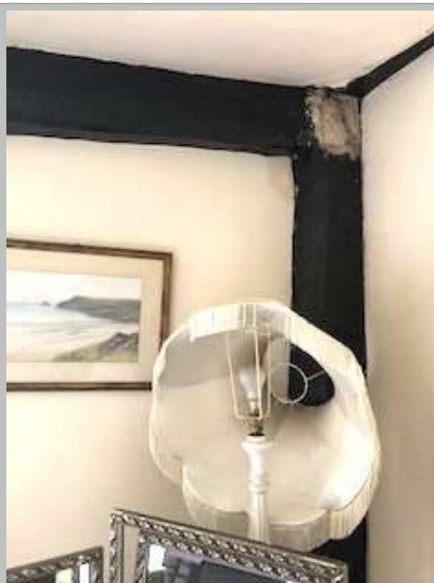
Plate 18. Beams and posts in bedroom NB damage at junction
