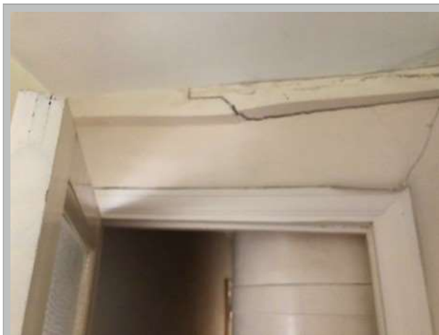
Plate 1a. Deflected structural timber beam
