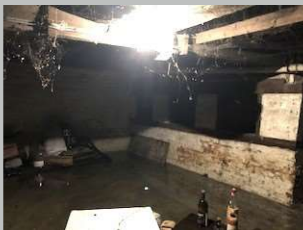
Plate 1b. Standing water in basement
